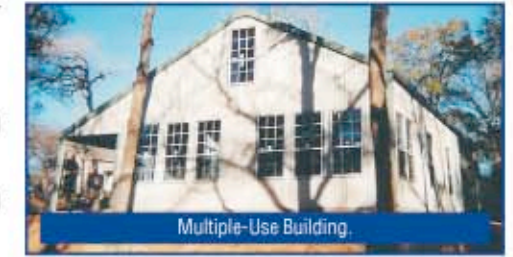
SBSI Arena Cover Built To Match Existing Building.
